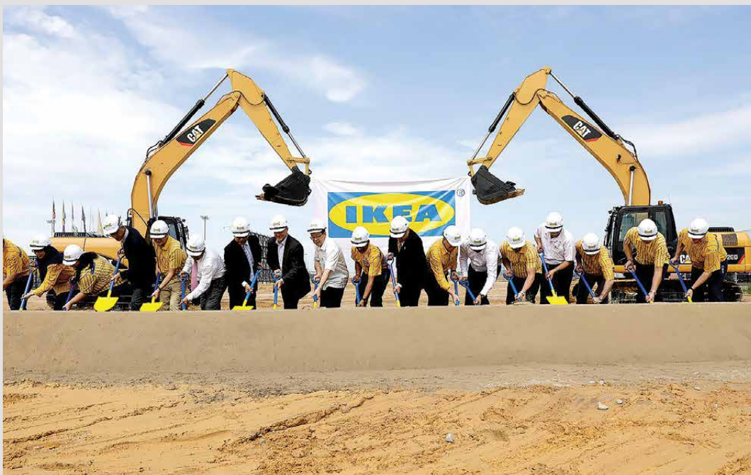
The first IKEA store in the Northern Region of Malaysia breaks ground at Aspen Vision City, Batu Kawan, Penang
